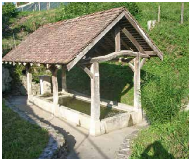
Wash-house of Villeneuve d'Uriage
